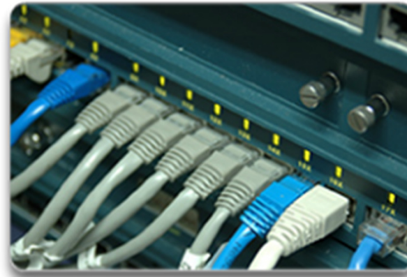
Cables must be connected correctly.
