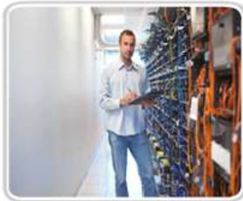
Installations must be inspected for damage.
